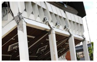
Fig 2 – Load path failure
