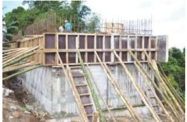
Construction of the tank (as of November 2015)
