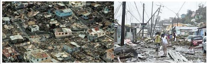
Figure 4. Roads in the capital of Roseau littered with structural debris, damaged vegetation and downed power lines.
